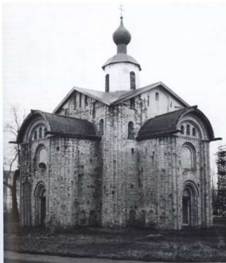
Figure 39. Church of St. Paraskeva Piatnitsa on the Marketplace, Novgorod. 1207, with extensive modifications in the fourteenth and sixteenth centuries. Partly reconstructed in the 1960s. (N 3-14)
